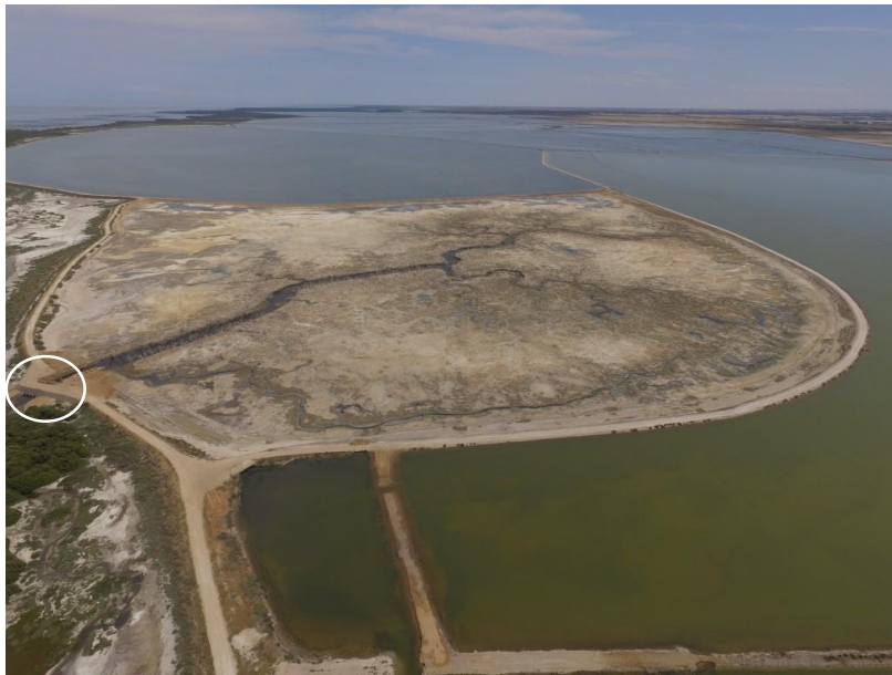
Figure 1. The trial pond XB8A of the Dry Creek salt field north of Adelaide, showing adjacent ponds with hypersaline water still operated under a holding pattern, and the mangrove/saltmarsh coastline on the left. The tidal gate installed as project activity can be seen where the creek passes through the levy bank. Photo taken at low tide several months after re-connection of the pond. Photo credit: Department of Environment and Water.
